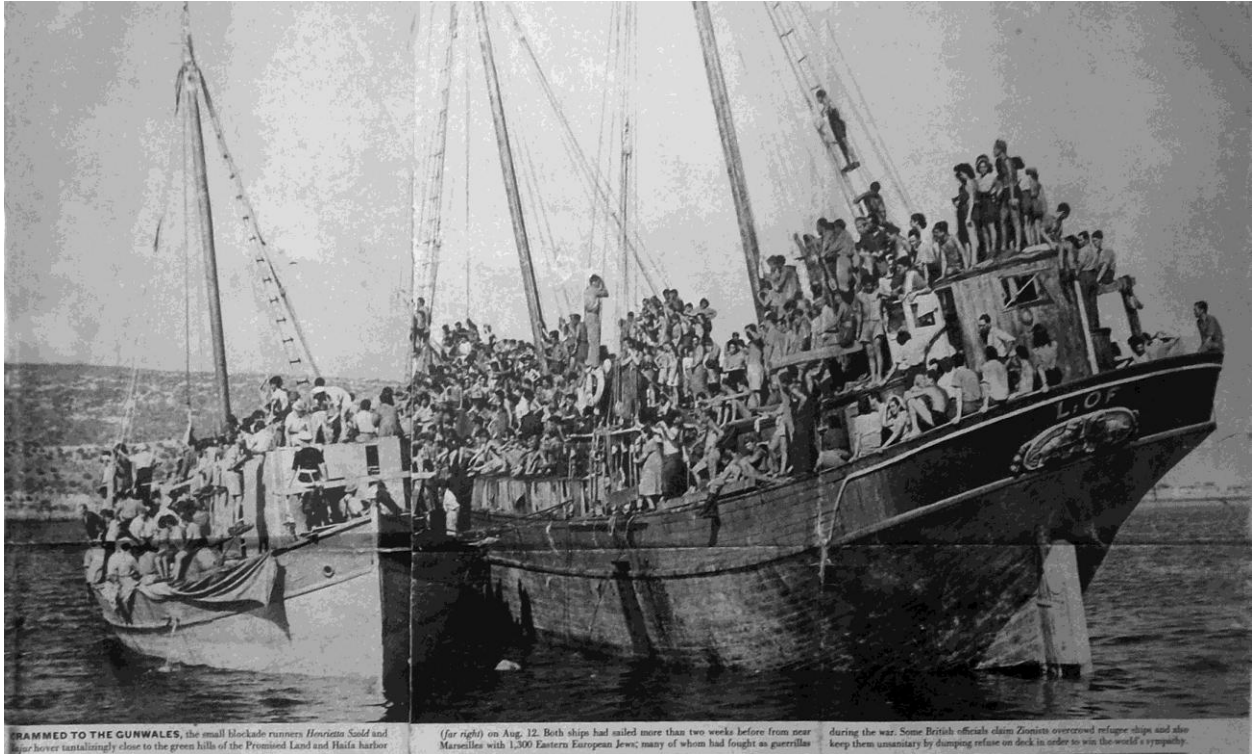
TRAPPED TO THE GUNWALES , the small blockade runners Hevriata and L.O.F. hover tantalizingly close to the green hills of the Promised Land and Haifa harbor
